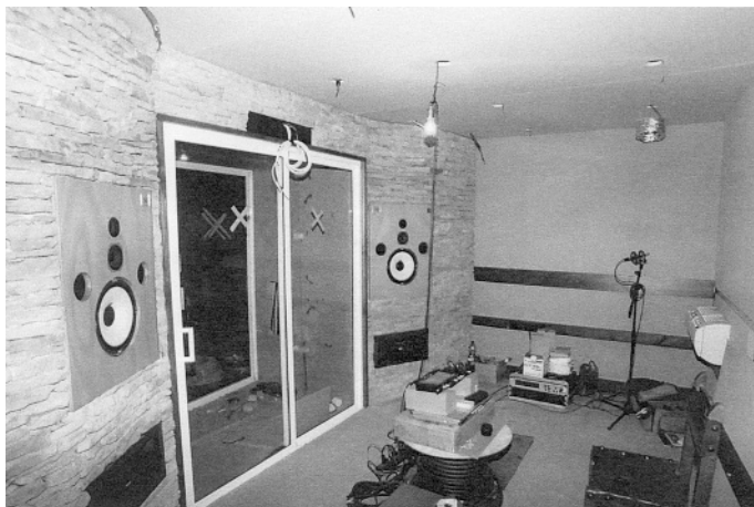
Figure 8.9 A small control room, under construction in Ubeda, Spain, with a miniaturised Reflexion Arts 240c system. The cabinets are large, to allow a generous and fast low frequency response, but the drivers form a compact group to minimise the geometrical near-field problems at short listening distances. The rear wall, side walls and ceiling are highly absorbent behind their fabric coverings
