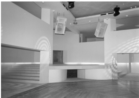
Figure 12.18 A concrete horn, under the stage, loads a cabinet with four 18 inch (450 mm) low frequency drivers. The response is essentially flat down to 20 Hz, and 120 dBC on the dance-floor is achieved with ease and reliability. The mouth size is 4 m × 1 m
