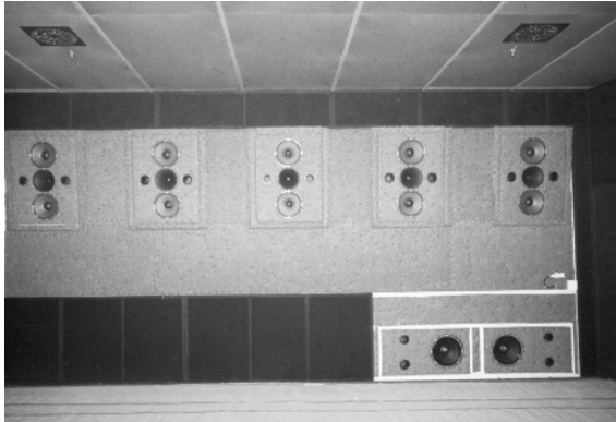
Figure 12.8 A cinema studio monitor wall for Sony SDDS 7.1 surround
